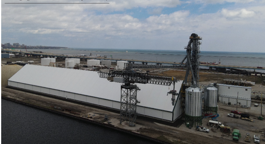
DeLong Agricultural Maritime Export Facility
